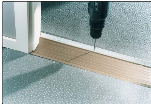
Fitting with the help of the drill template.
